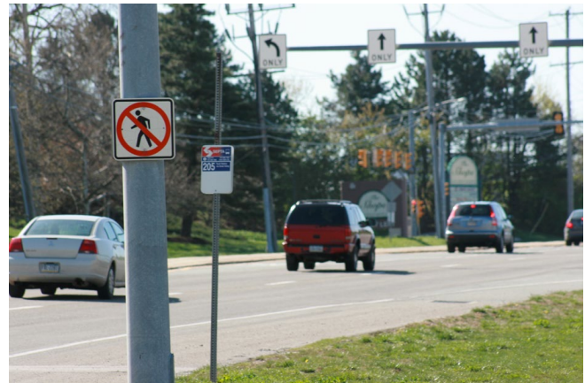
Substandard pedestrian environment for a bus stop.
