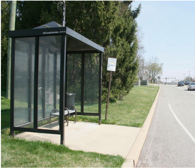
Bus shelter with no pedestrian connections.
